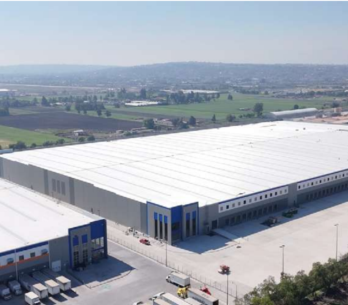
Parque Industrial Danhos Palomas (Phase II) The second phase of the Danhos Parque Industrial Palomas property, a 110,000 m² build-to-suit complex that will be developed in three phases: the first, 65,000 m², is under construction and will be delivered in December 2026.
